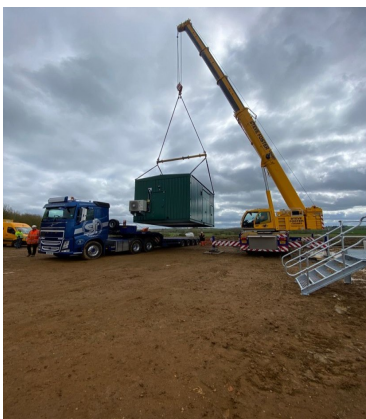
Landing of containerised 33kV Substation
