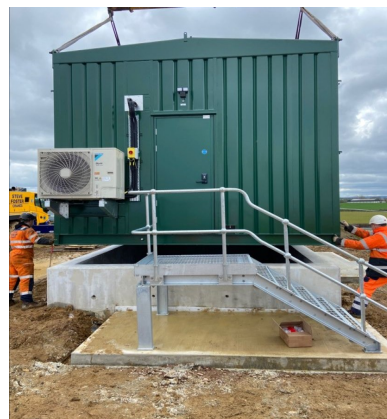
Landing of containerised 33kV Substation
