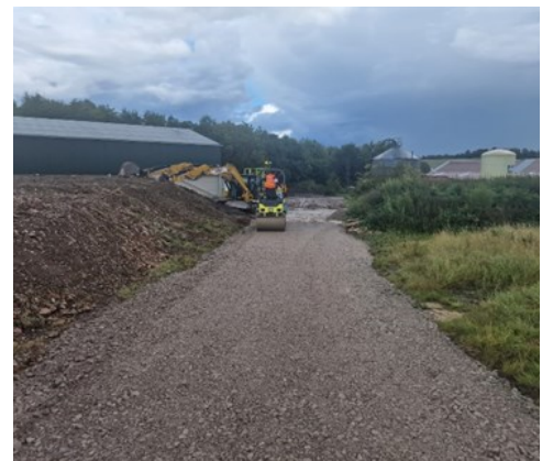
Construction of unmade access road to substation
