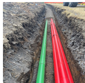
33kV Cable Laying
